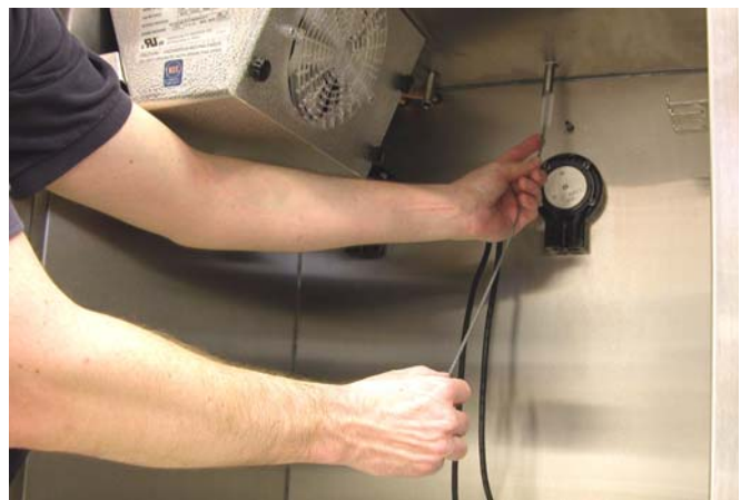
Figure 25. Cleaning Feed Tube
